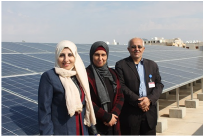
Head teacher Amine Alwneh (left) in front of the solar panels on Hay Al-Karamah School in Irbid.
