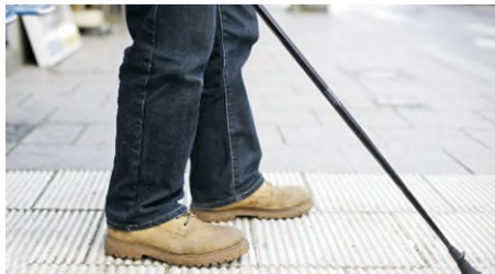
Ground surface indicators also make it possible for visually impaired people to find their way on public transport.
