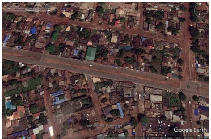
4.3.5.4: Google Earth image of the western part of the road after the end of the project in 2018
